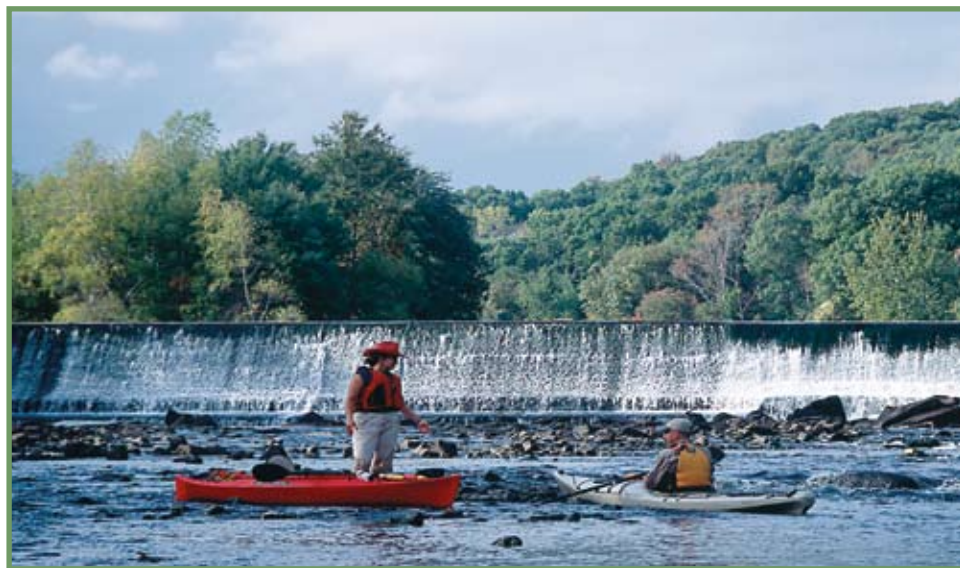
Below the Albion Dam on the Blackstone River.
